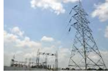
Transmission Line EPC
