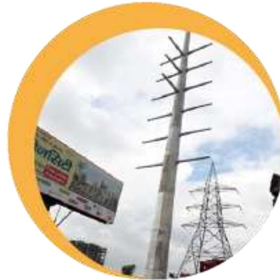
220 kV M/C pole with aux cross-arms
