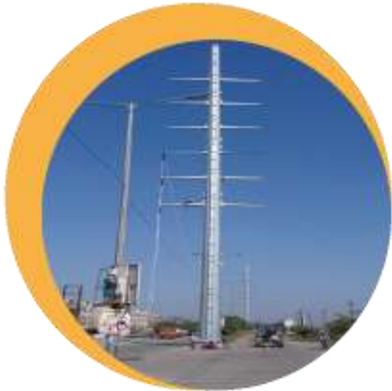
Base plate pole on median
