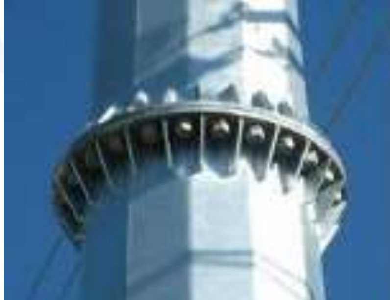
FLANGE TYPE JOINT
